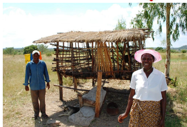
Raised from ground poles and thatched goat housing
