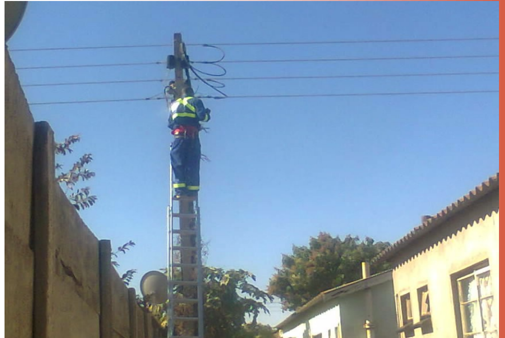
A solarhart technician at work installing electricity prepaid meters in Zengeza 1 recently.
