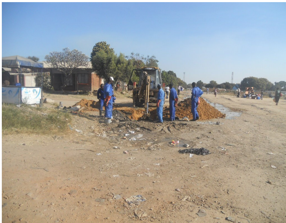
Municipality workers and their machinery at the corner of Rufaro and Hombarume
