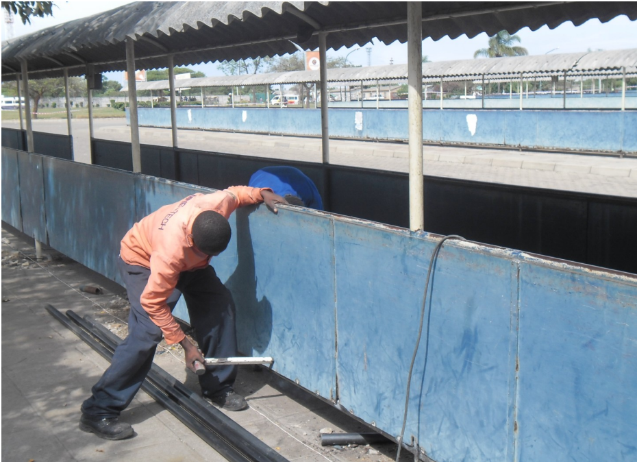
An employee of Ofaclaim renovating Chitungwiza town centre bus terminus.
