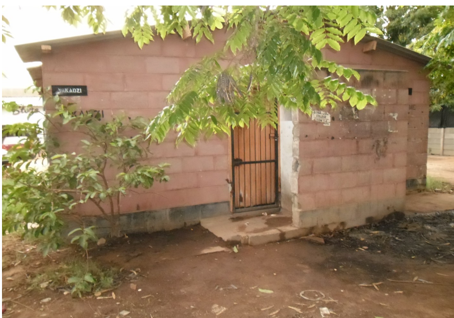
A public toilet at Zengeza 5 shopping centre.
