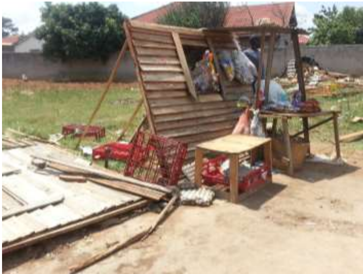
One vendor continues his business at the demolition site
