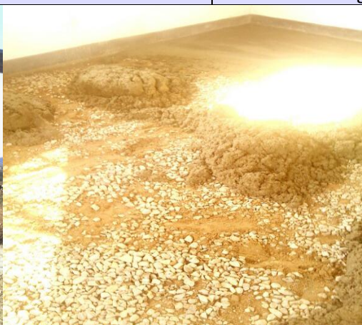
Poor workmanship at the fast tracked Anjin built Houses at Arda Transau causing walls to crack and floors to disintegrate
