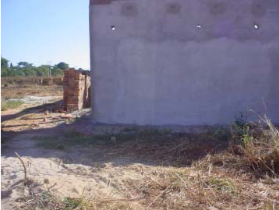
Plate 6: Another huge House under construction at Aspindale
