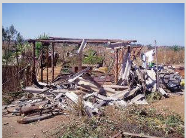
Demolished house at Hatcliffe.
