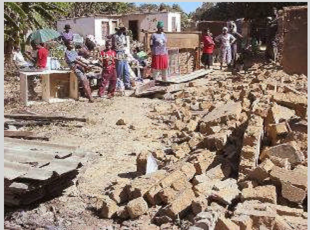
Family Demolishes own house in Epworth, Harare.
