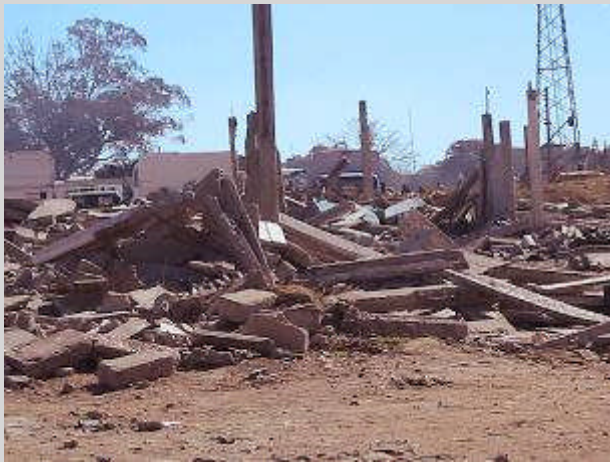
Market stalls demolished in Mbare, Harare.
