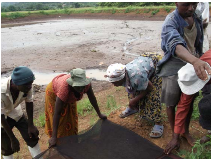
Hands on IAASL: Beneficiaries preparing an outlet screen for their overnight storage facility at Magudu Scheme in Ward 29, Masvingo District
