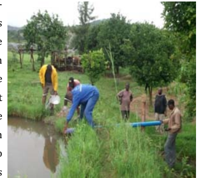
IAASL Beneficiaries Fitting an Overflow Pipe on a Fish Pond
