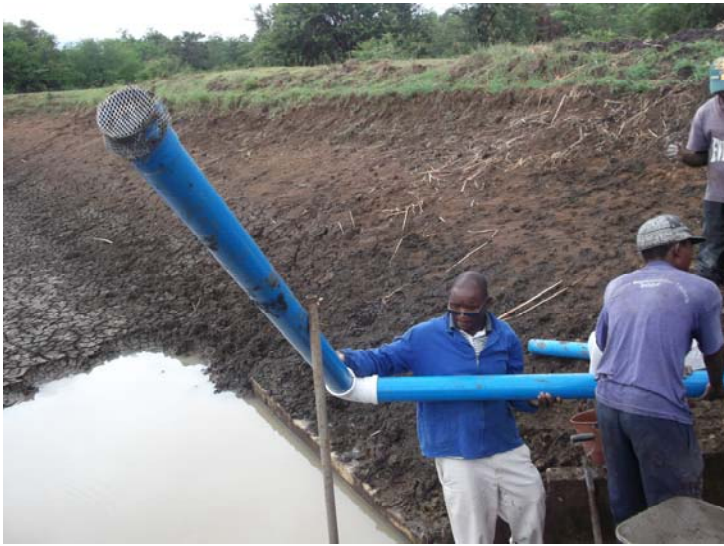
An Aquaculture Zimbabwe Field Officer demonstrating how to install a drainage pipe at Chisase Ponds in Ward 30, Masvingo District
