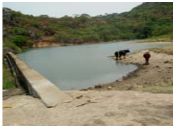
A great potential site identified
